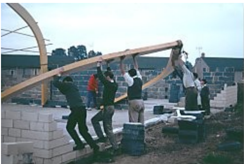
Raising the arches
