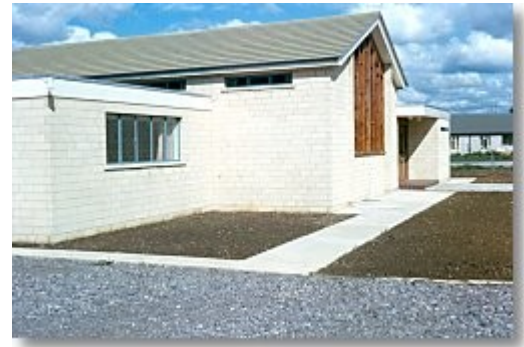
The newly completed chapel
