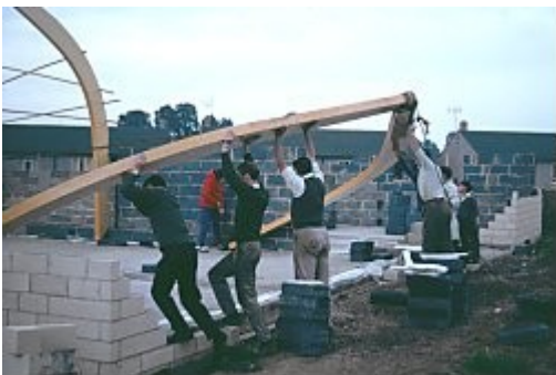
Raising the arches
