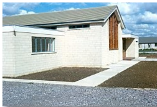
The newly completed chapel
